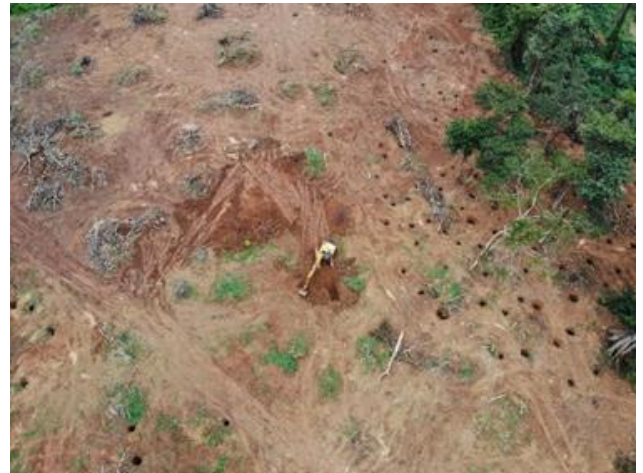
Backfilling old artisanal mine shafts in the TSF area
