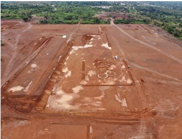
Plant site CIL ring beams excavation
