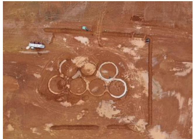
CIL ring beam blinding
