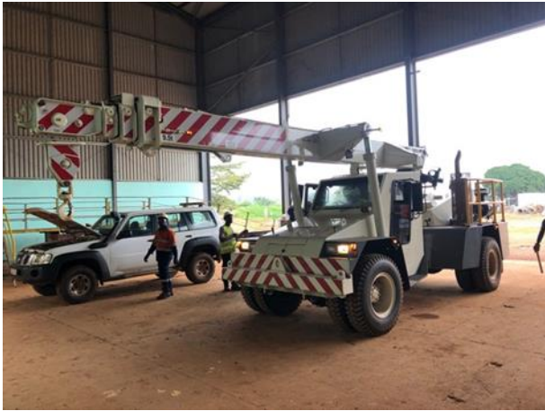
Franna Crane delivered to site
