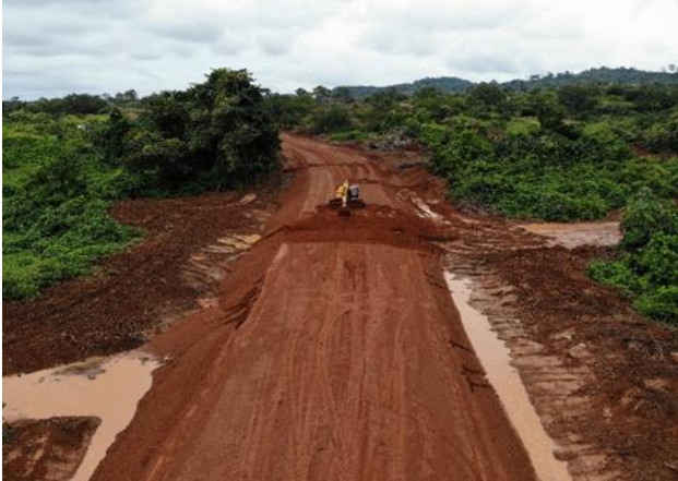
Fence line Road culvert installation
