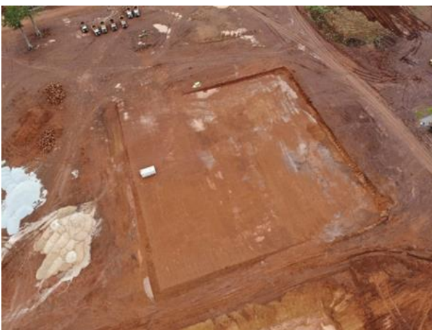
Switchyard building pad
