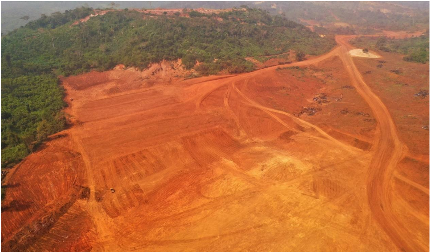
Tailings Storage Facility – Stage 1 site
