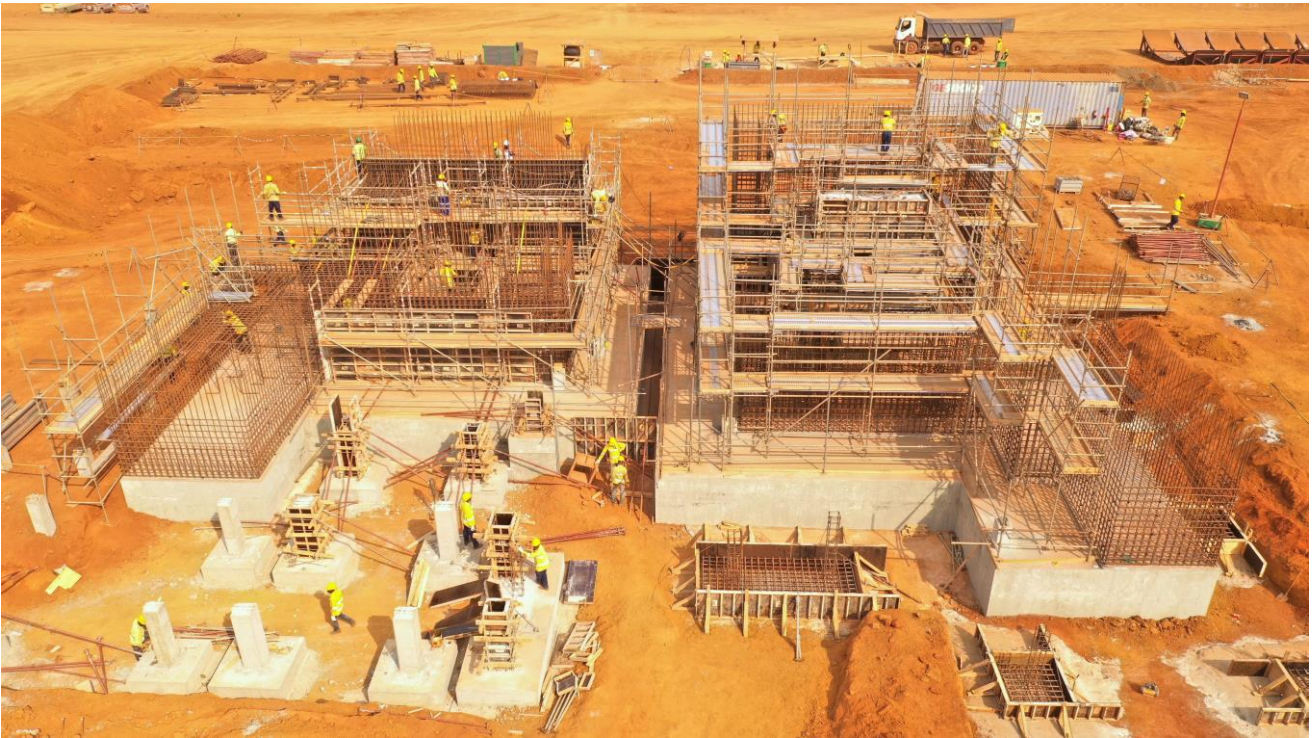
Ball and Sag mill foundations and support structure
