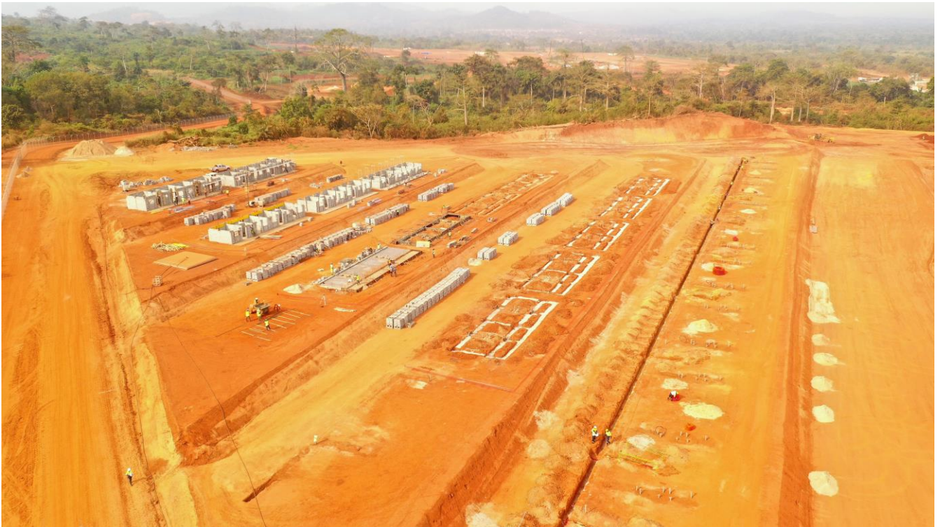
Aerial view of Permanent Camp
