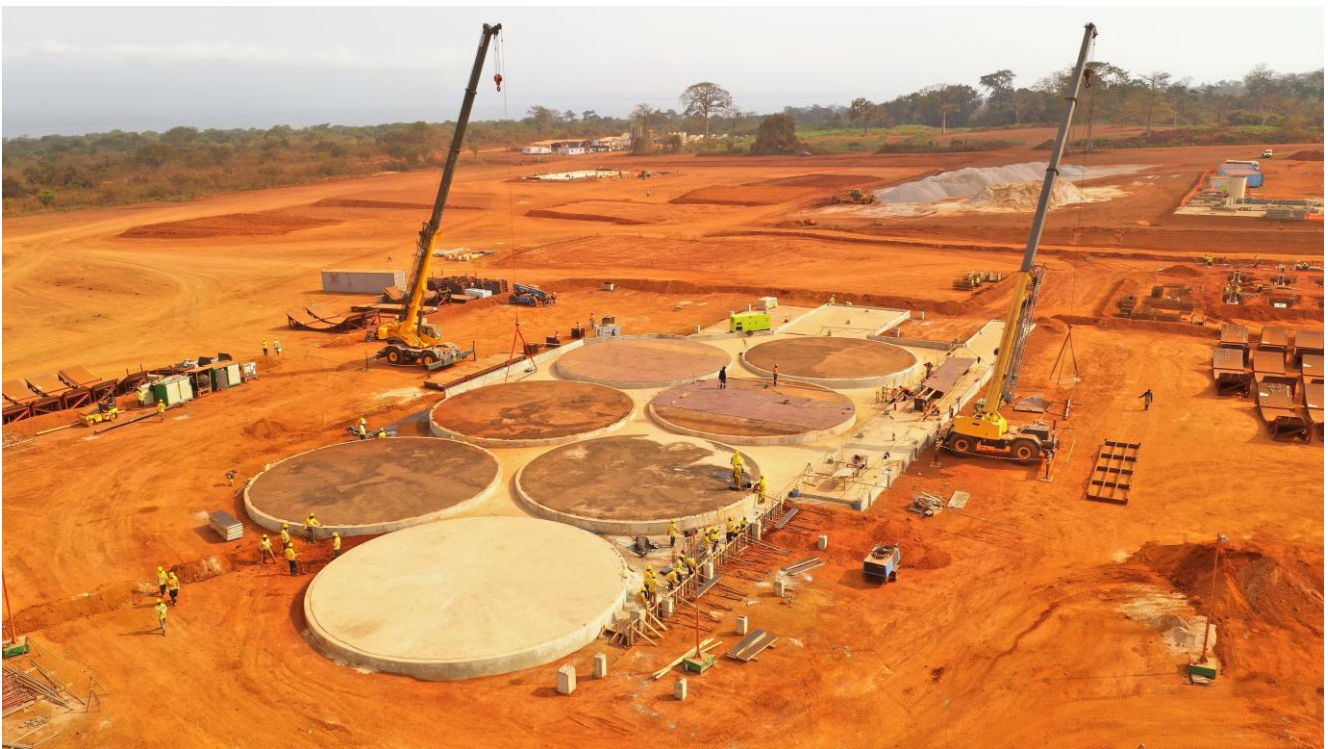
CIL Tank foundations
