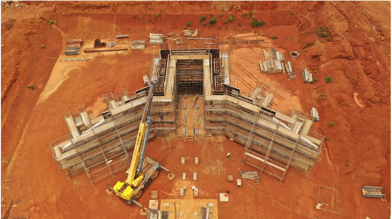
Primary Crusher Foundations
