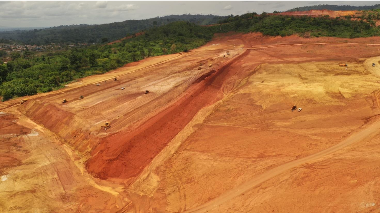
Tailings Storage Facility Site Overview – West Embankment
