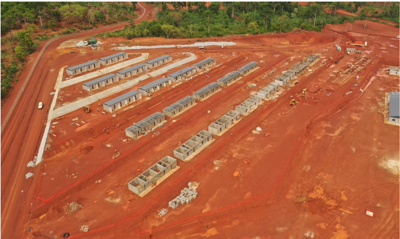
Aerial view of Permanent Camp
