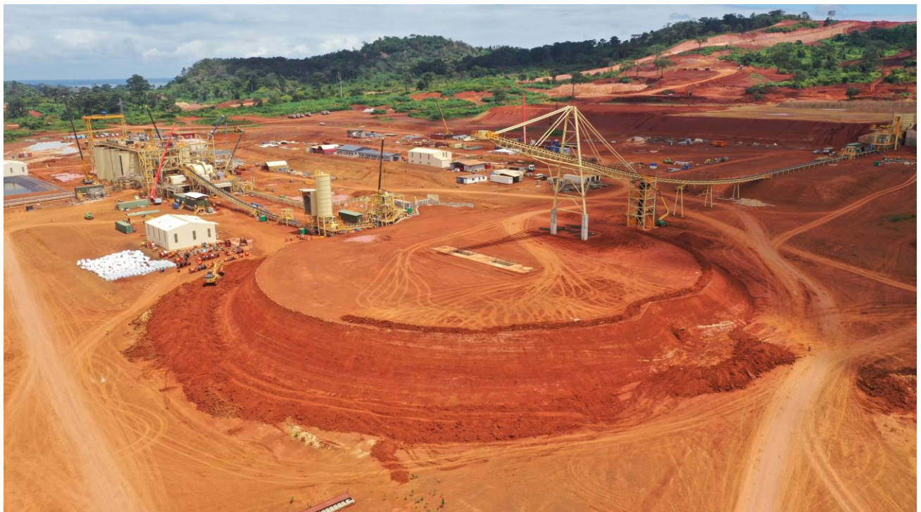
Crushed Ore Stockpile feed conveyor
